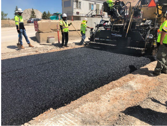
Figure 1 June 2021 Test Strip, Staker Parson Facility
